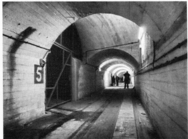
Side passage off the main tunnel at St Aubin – constructed as Ho5. Parallel 60cm rail tracks can be made out.
